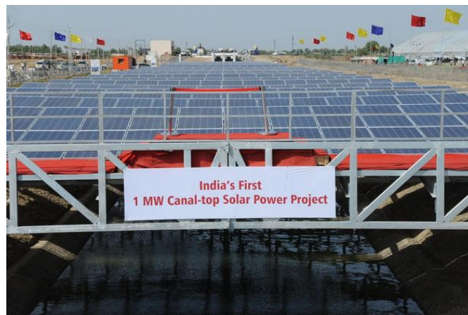
Figure 2. The solar panels on the Narmada canal. (Source: Google images).
